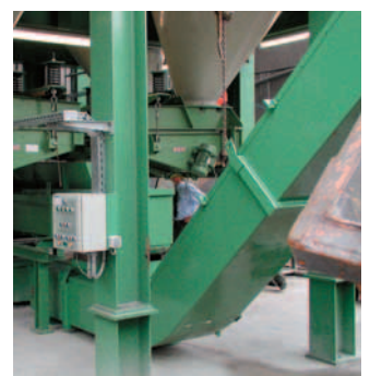
■ Scraper conveyor under a hopper system for aluminium chips
